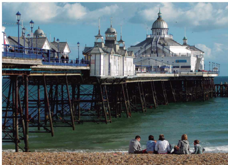
Old zinc roofs on Eastbourne Pier, England.
