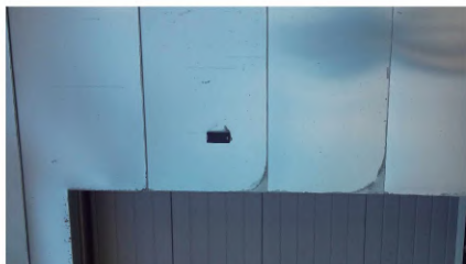
Partial removal of protective film causing differential weathering on natural zinc. These differences will weather-out over time
