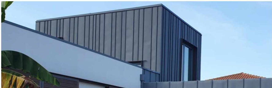
Housing development. Standing seam in zinc.
