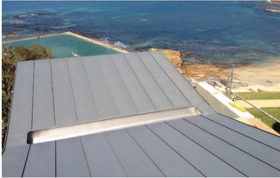
Frequently rain-washed areas do not allow salt deposits to build – elZinc Slate at Fairlight, Sydney
