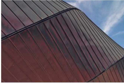
Double lock standing seam in copper
