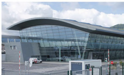
Cruise liner terminal in Getxo, Bilbao, Spain, in elZinc Natural. Left photo taken three months after opening, Right photo 18 months later.
